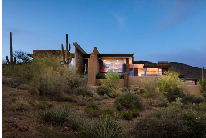
Exhibit 4. Low-profile building minimizes visual impact.
